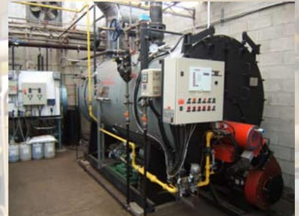
Autoflame linkageless controls with variable speed drives and independent servomotors adjust the air-to-fuel ratio and the burner firing rate to precisely match the required temperature or pressure setting of the boiler. Optimum combustion efficiency is constantly maintained regardless of load and environmental changes.
