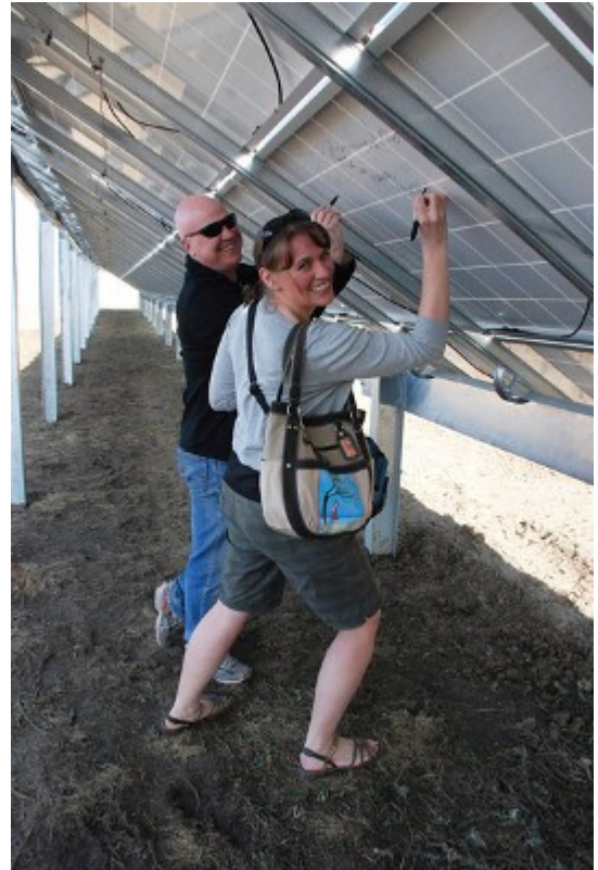
Customers signing their panels in Clean Energy Collective's Boulder Cowdery Meadows Solar Array, Boulder, Colorado.
