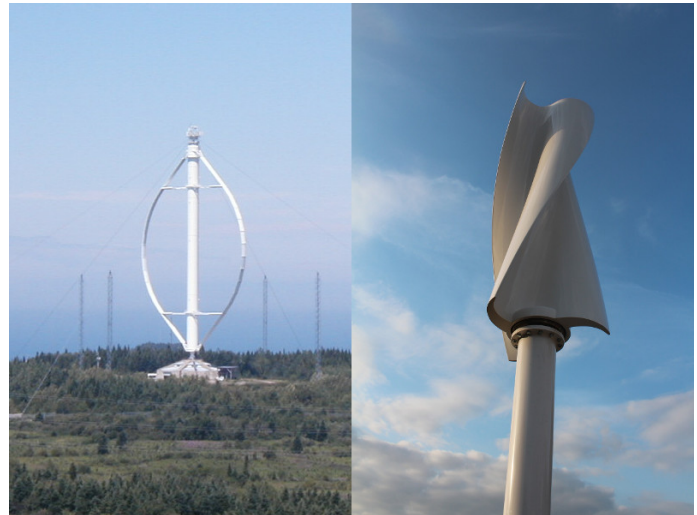
A Darrieus wind turbine (left), and a Savonius wind turbine (right) Darrieus photo CC BY-SA 3.0 by Guillaume Paumier . Savonius photo CC 0 by Bernd Wolf .
